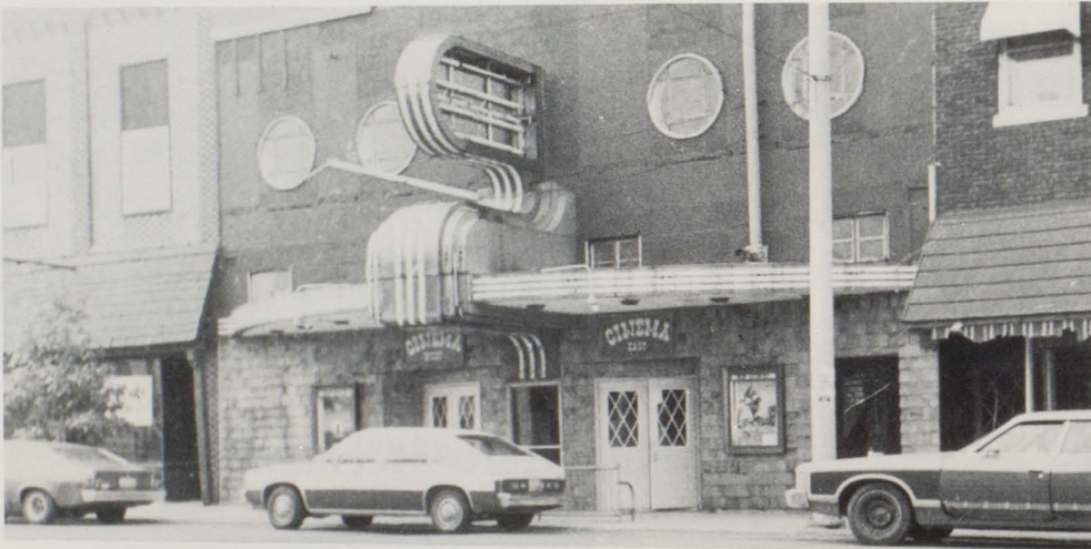
The Elwood theatre has been at its present site on Main Street for several years. But, this year it was renovated and changed into a twin cinema.
