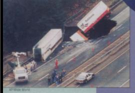
Days of abnormally heavy rains in November undermine the roadbed of Oregon's Interstate 5, creating a 40-foot-deep sinkhole, into which two semitrailer trucks tumble.
