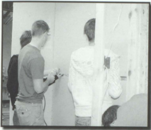
Shane Stotts and Austin Crouch construct a wall.
